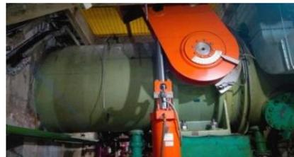
Gambar 5. Pipa Pesat PLTA Way Besai
