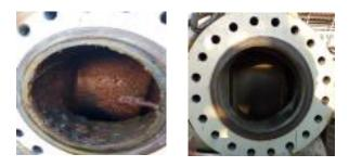
Before Chemical Injection After Chemical Injection Picture-2: Before and After Chemical Cleaning injection.
